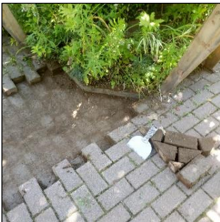
Resetting the walkway pavers
