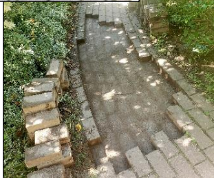
Resetting the walkway pavers
